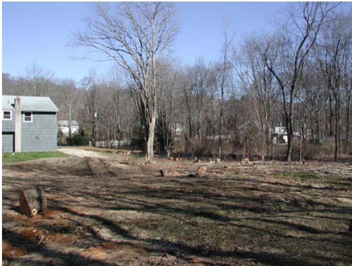
View of designated wetland area from back yard looking toward house (left). Tree cutting ended at visible water (right). Channel will be enhanced, and will carry flow from under driveway.
