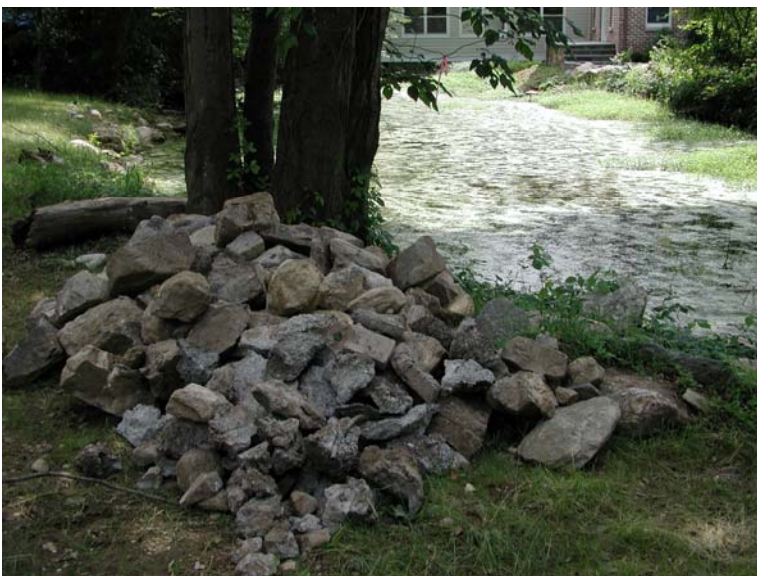
Fill brought on site post orders.
