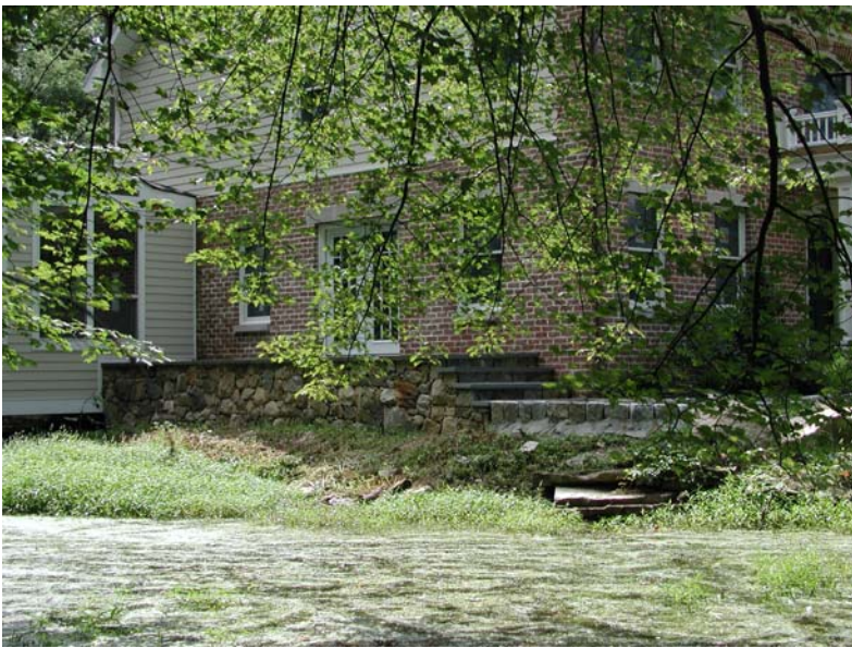
Newly constructed terrace and walkway along pond sans approval.
